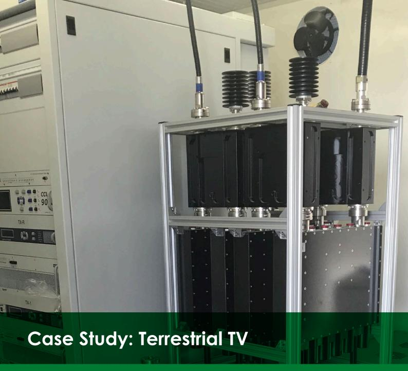
Enabling 49 additional Digital TV channels in PNG via a new DVB-T2 Transmitter
